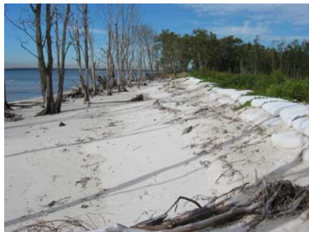
Above, the "great wall of Towra" constructed to slow the erosion of Towra Beach, caused by development within Botany Bay.
